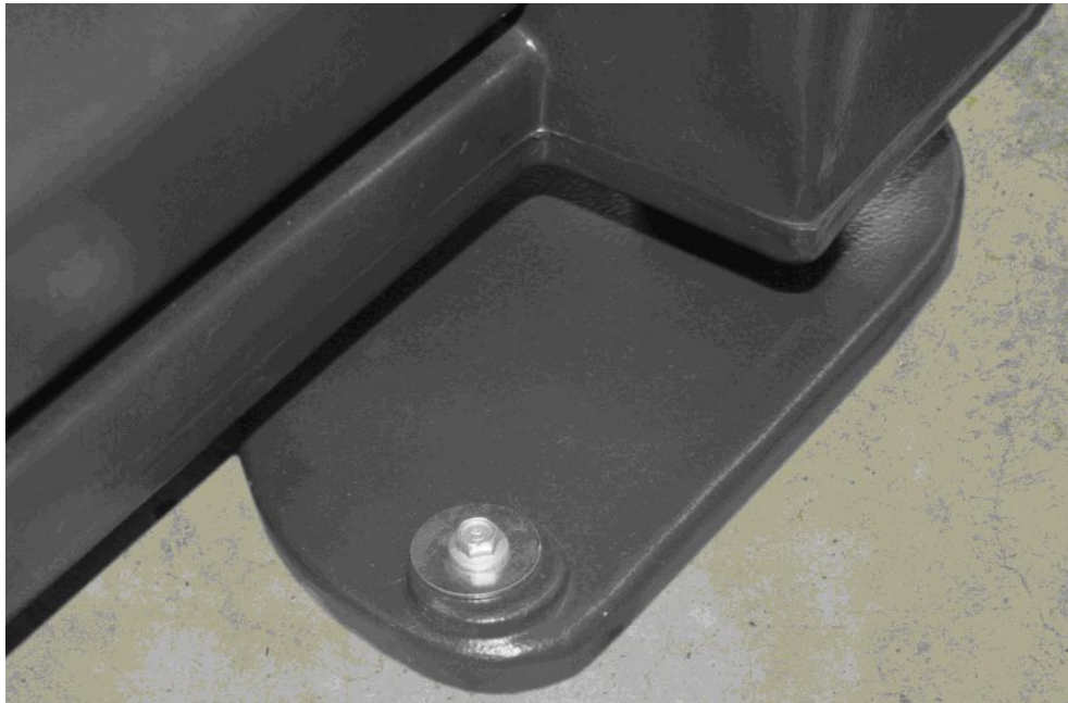
Figure 7. Fixing to pad.
